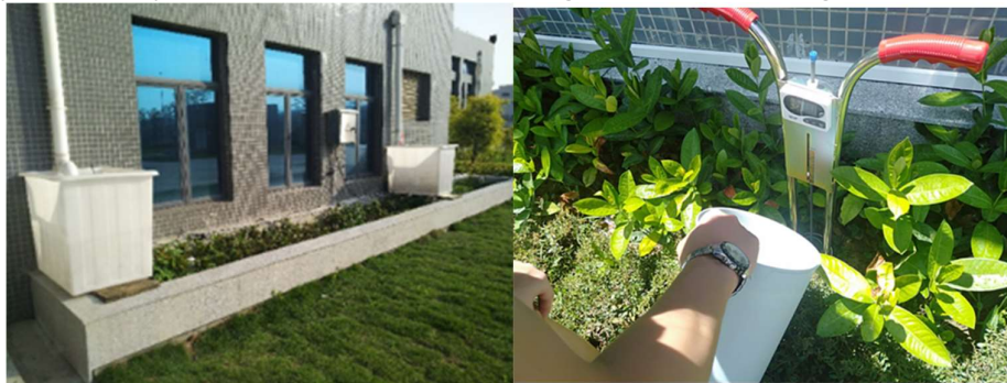
Figure 1 The bioretention cell built for modelling development, calibration and validation.
