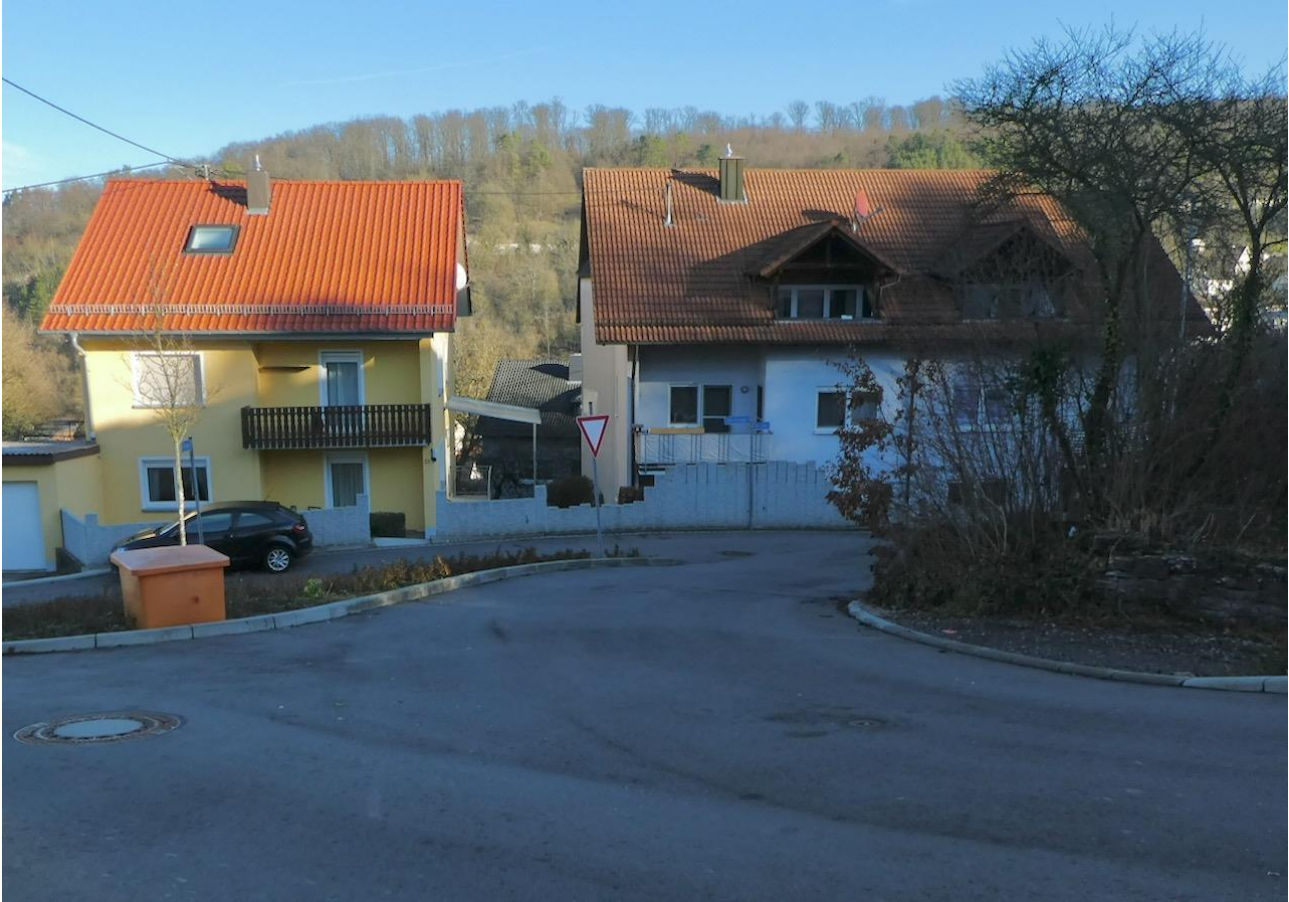
Figure 1: Example of a house protection (see the wall in different heights as function of the safety level required) in a municipality after a damage caused by high downhill flow on the street
